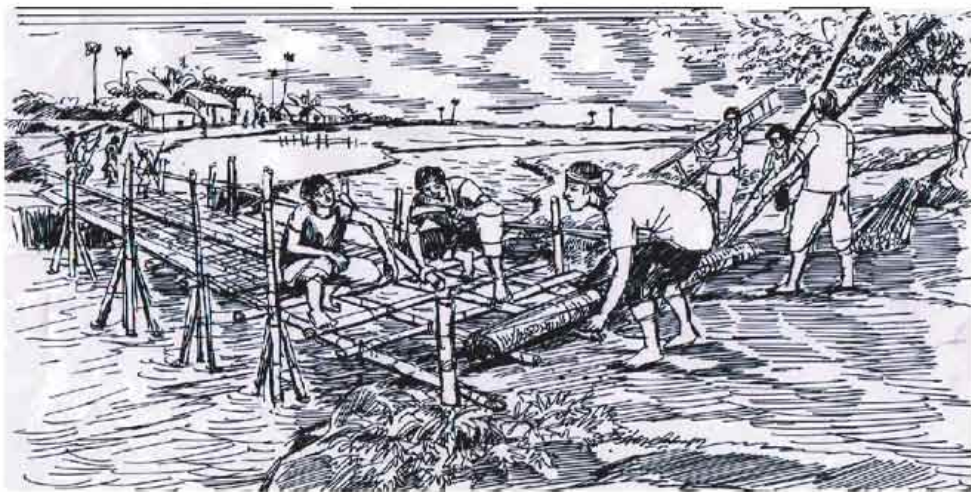
Youths are repairing the bridge.
