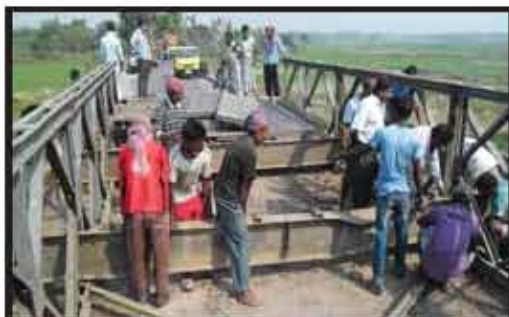
The workers are repairing the bridge.
